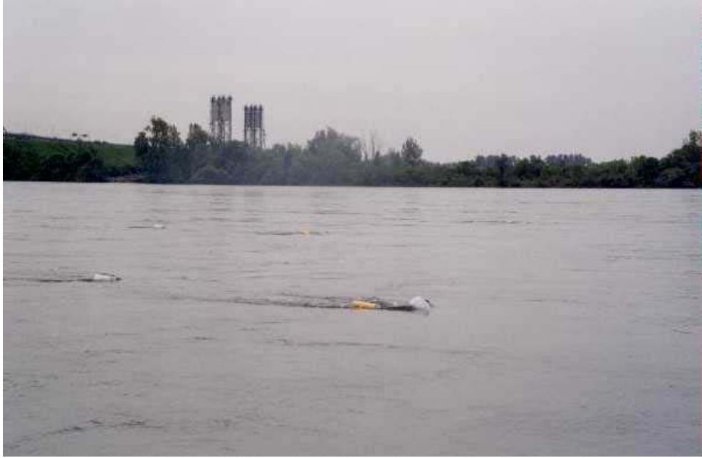
Photo 3. Systematic installation of parpens, upstream portion of the Lachine Rapids, spring of 2002. The distance between the first two floats was set so that for an observer standing some twenty metres away, the space that separates the parpens is completely covered by the person's thumb, thereby facilitating the estimate of distances on the body of water.
