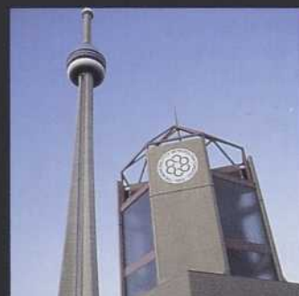
John Street pumping station
