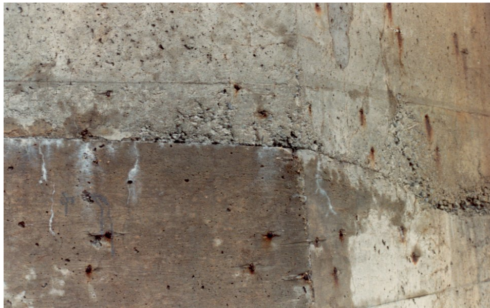
Photo 4.2-6 a) Joint froid
