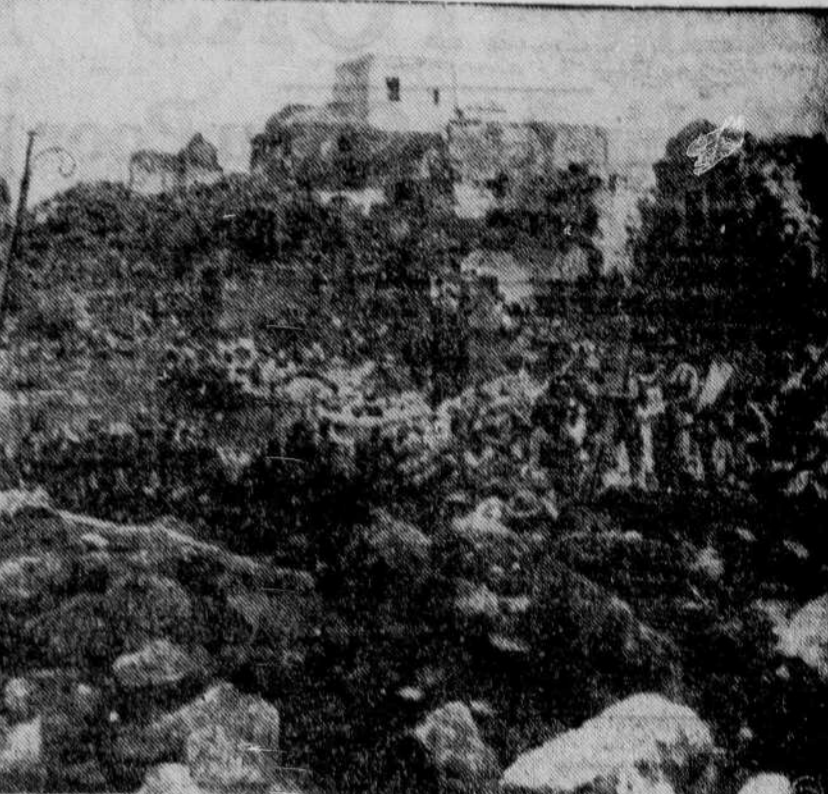
Ragged skeletons of blasted buildings and a terrain covered with rubble was the look of Pantelleria when British troops took possession of the Italian island stronghold after one of the war's most intensive air and sea bombardments.
