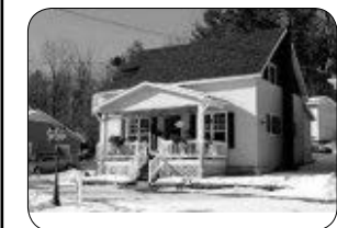
93 GREENLAY S, WINDSOR COTTAGE 3 CC, GRAND TERRAIN.
