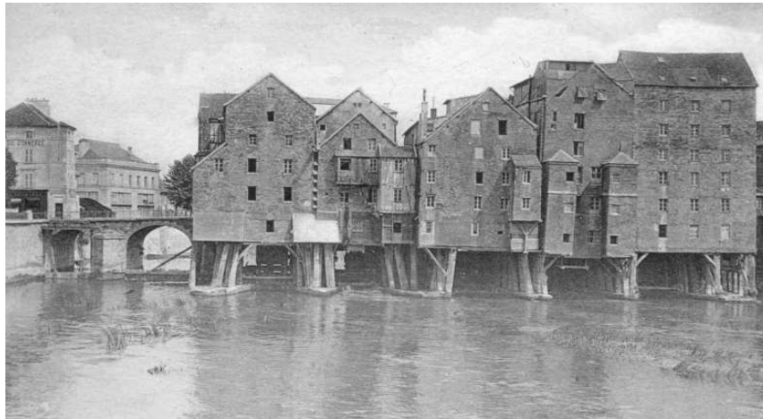
Rue Vieux Moulins circa 1920. Several mill buildings, constructed in the sixteenth century, sit atop the Rue Vieux Moulins with the river running beneath. The flow of water was important for the operation of machinery for grinding wheat, a traditional milling activity. Waterpower was also used in founding and to run the fulling machines necessary to the trade of Estienne Charron. The building he rented in 1573 may have been one of these.
