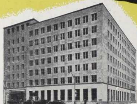
Bell Telephone Co. of Canada, Toronto Mathers & Haldenby, Architectes
