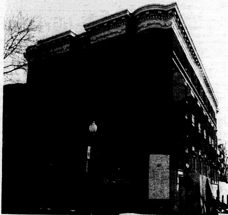
Work is under way to convert the former Western Apartments building at Olivier avenue and de Maisonneuve boulevard into Manoir Olivier, a 16-unit condominium building.
