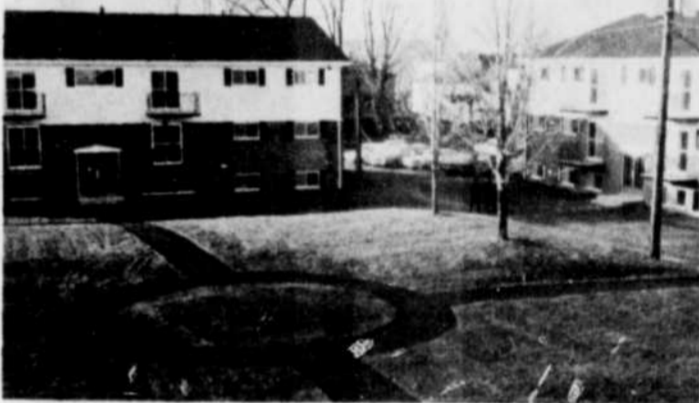
PROJECT CAROLINE READY FOR OCCUPANTS
